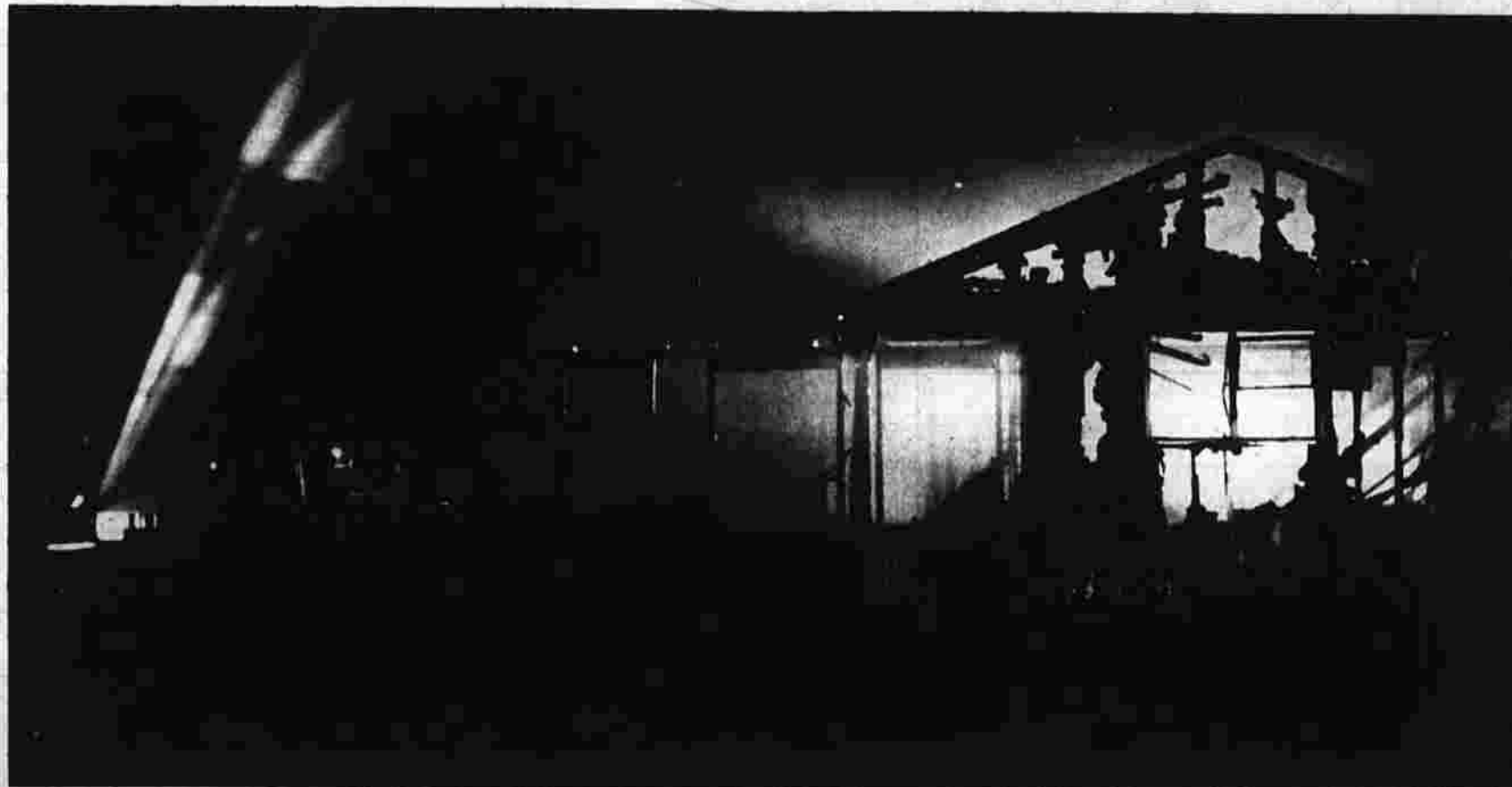
Light from the fire shines through stream of water shooting onto remains of a house, under constructions, at Flagg and Scott Drs. (Herald photo by Pinto)
